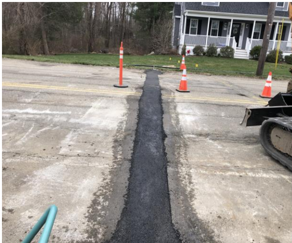
Photo 3: Paved Trench Crossing on Auburn Street
