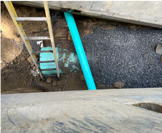
Photo 3: Replaced Sewer Service at #703 Auburn Street
