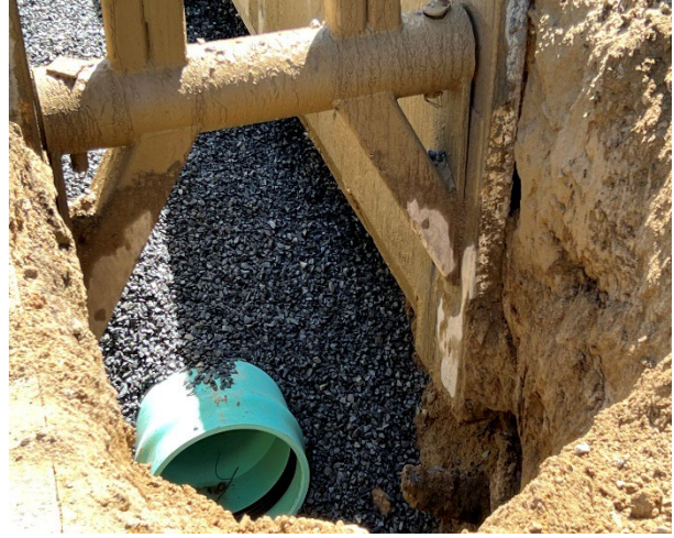
Photo 2: Crushed Stone Placed After Pipe Installation
