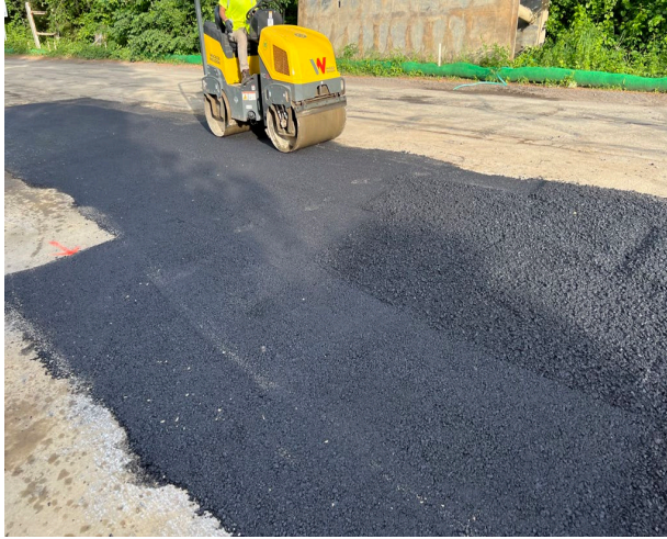
Photo 1: Trench Compaction After Paving
