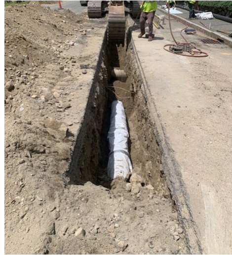
Photo 2: Installation of 12" DI Water Main Under Existing Drain
