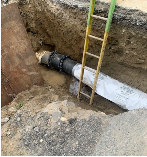
Photo 1: New Solid Sleeve Connection from New 12" DI to Existing 12" DI Pipe
