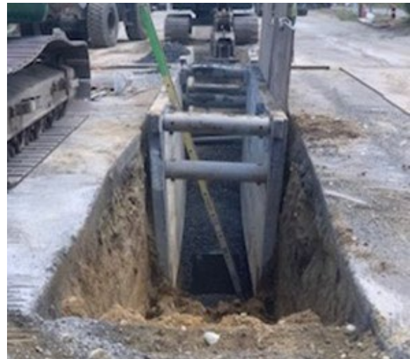
Photo 3: Trench Box for New 20-Inch PVC Sewer Force Main
