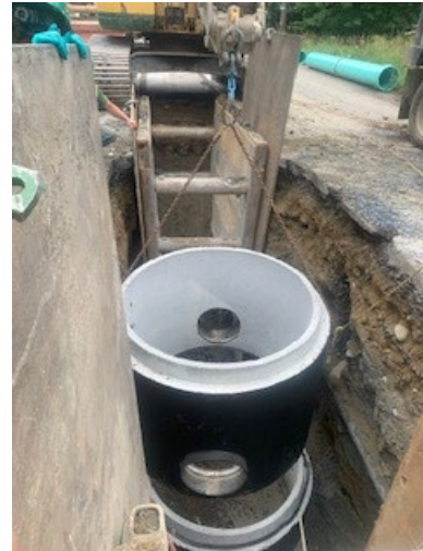
Photo 3: Installation of 6-foot Cleanout Sewer Manhole on Auburn Street
