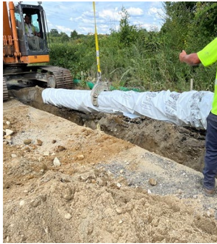
Photo 1: Installation of 12-inch DI Water Main on Auburn Street
