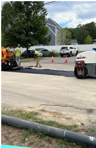
Photo 2: Temporary Paving of the Sewer Trench on Auburn Street
