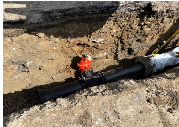
Photo 1: Installation of 12-inch DI Water Main on Auburn Street
