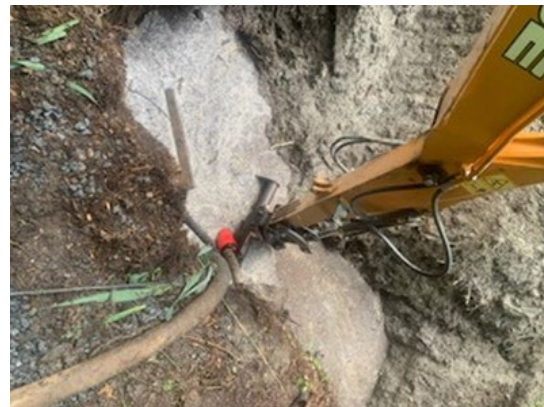
Photo 3: Exploratory Test Pit in Cross-Country Easement to Locate Existing Utilities
