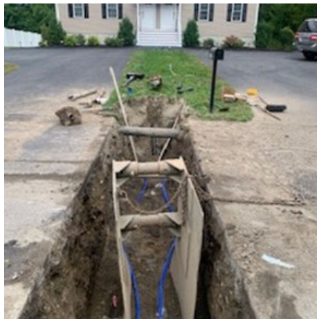
Photo 1: Installation of 1-inch Water Services for #1045 and #1047 Auburn Street
