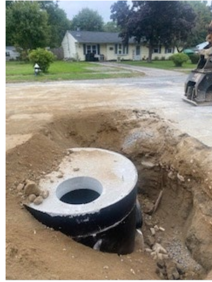
Photo 3: Terminus Manhole Installation on Southfield Dr
