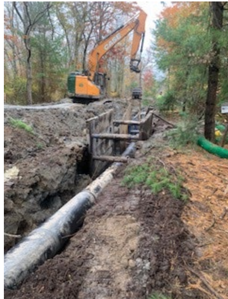
Photo 3: New Sewer Force Main Installation in Cross-Country Easement
