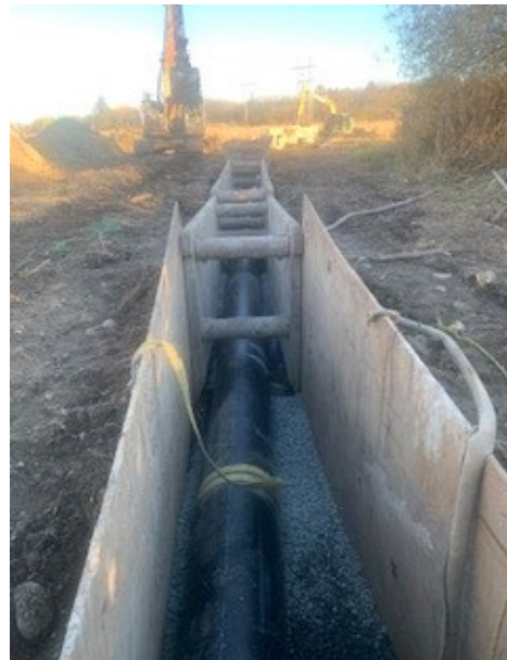
Photo 3: Installation of New 20-Inch Sewer Force Main in Cross-Country Easement
