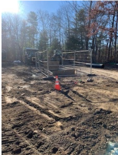
Photo 2: Work Zone Secured with Fencing near Meter Pit
