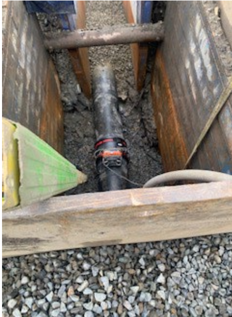
Photo 1: Trench Box Support for HDPE Force Main Installation
