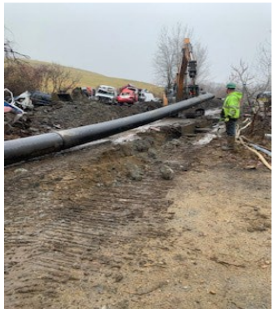
Photo 2: Lifting HDPE Pipe into Trench inside Junk Yard Easement
