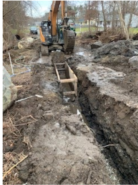
Photo 2: Trench Excavation in Landfill Easement
