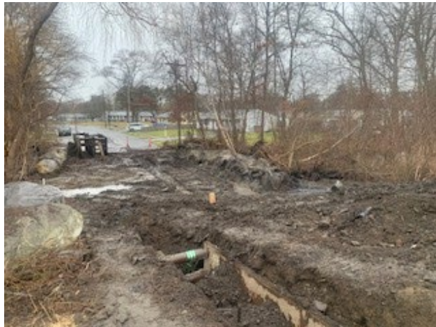
Photo 3: Backfill Restoration of Landfill Easement near Southfield Drive
