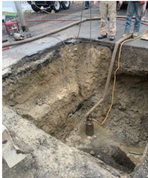
Photo 3: Dewatering of Excavation on Auburn Street
